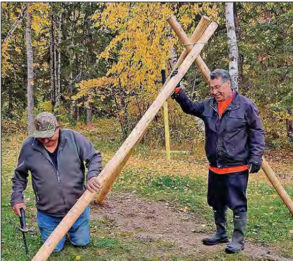
With a helping hand, Elzear Orr (kneeling) builds a meat drying rack at Wabasca Lions Campground, site of the Northland School Division's day camp.
